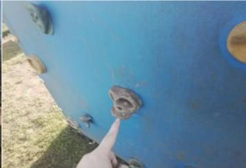
Finding: A number of handgrip fixing(s) have worked loose Action: Secure all loose fixings
