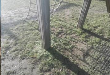
**Finding:** The timber stain is in poor condition
