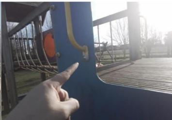
Finding: A number of barrier fixing(s) have worked loose
