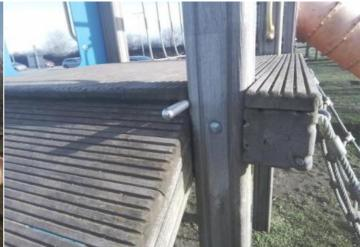
Finding: There is/are finger entrapment/s in the framework Action: Monitor - No remedial work recommended and the item fails to meet the requirements of BS EN 1176 Part 1 4.2.7.6 Entrapment of fingers
