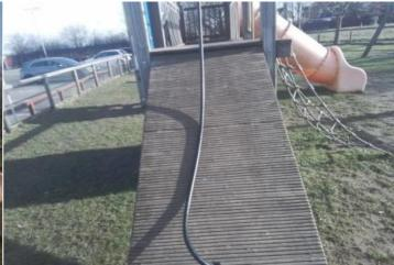
Finding: The chain connection cannot be inspected without Action: Dismantle the cover to inspect connection dismantling the cover
